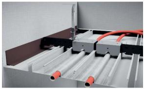
Progressive panel installation has to ensure a flawless ceiling design and an even levelled area – with sliding panels.
